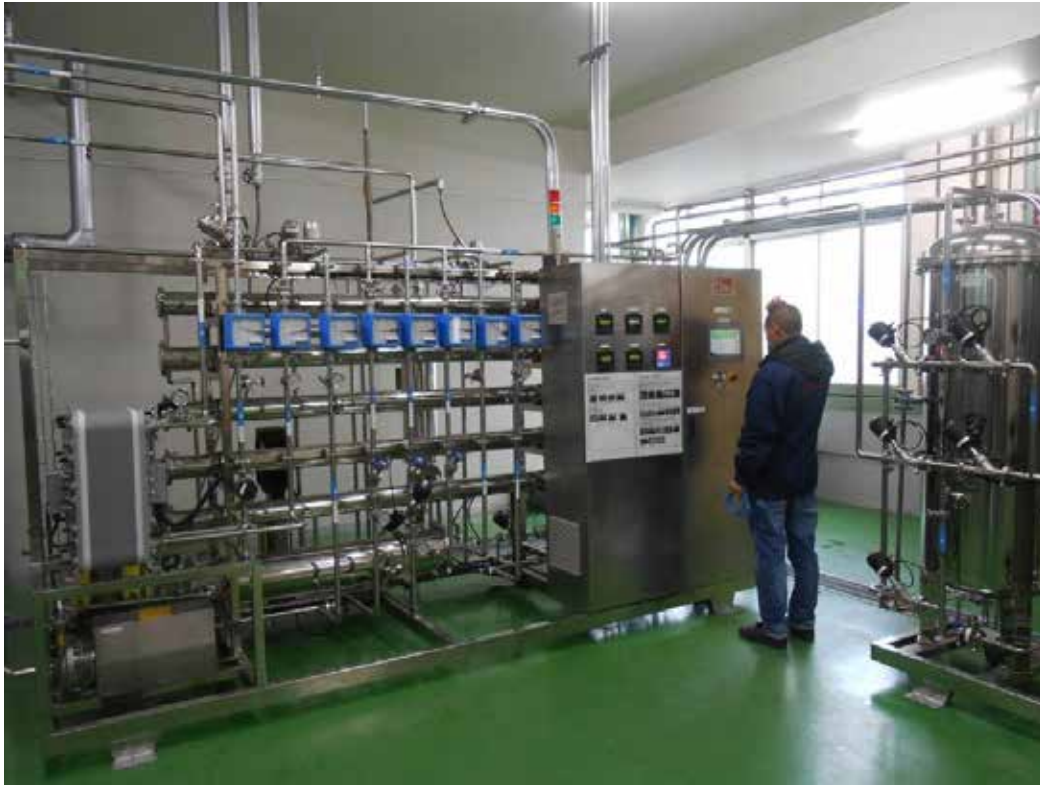
Highest Standard 2RO+EDI+UF System with PLC and Touch Screen Automatic Control System
